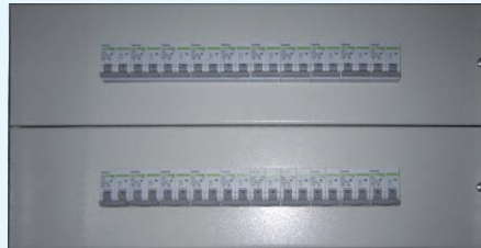
Miniature circuit breaker (MCB)
