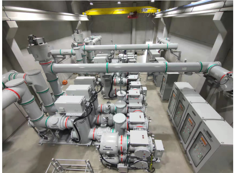
Compact Gas Insulated Switchgear (GIS) up to 145kV
